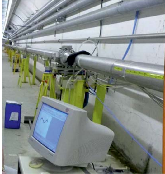
Fig. 2. The Transfer Tunnel general view in the experiment location area
