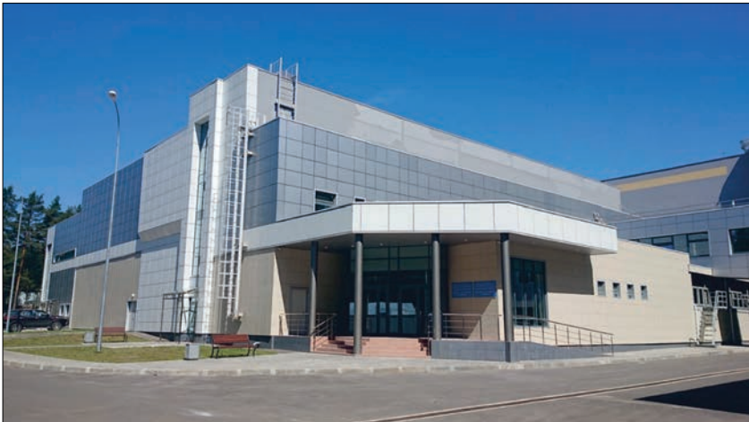
Building of the SHE Factory
