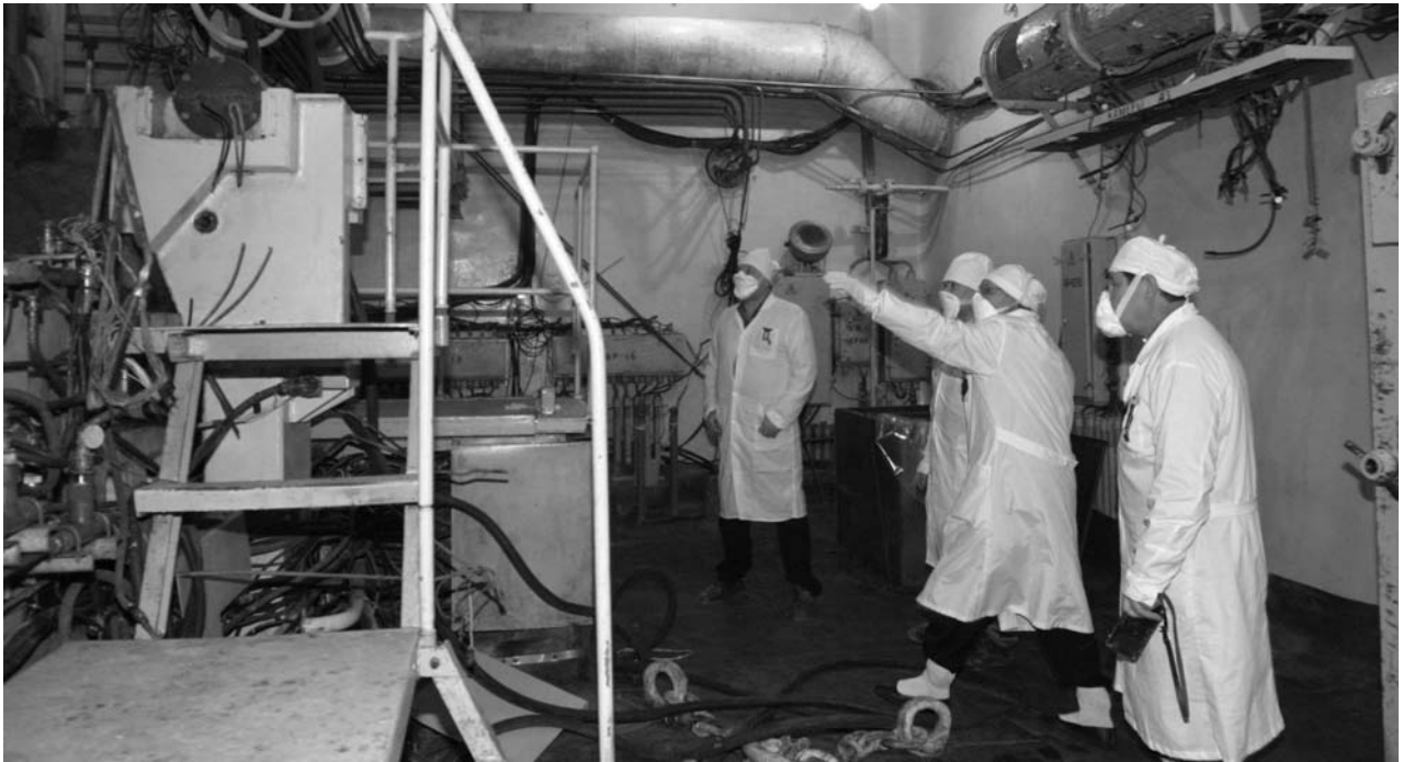
Frank Laboratory of Neutron Physics, October. IBR-30 dismantling
