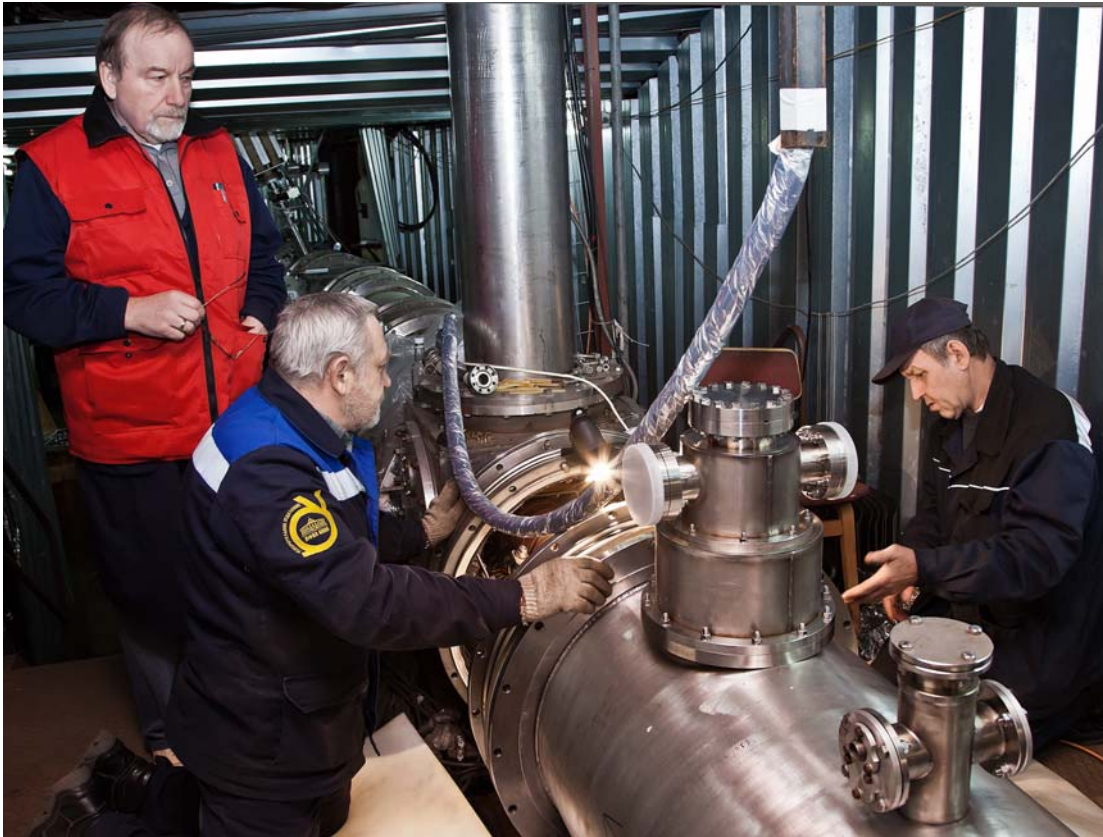
Veksler and Baldin Laboratory of High Energy Physics, 27 October. The final stage of installing the major elements of the stochastic cooling system for accelerated beams on the Nuclotron ring
